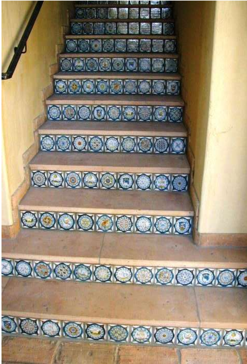
6”x 6” FAENTINI tiles used on stair risers. Painted in Blue and Brown colors on a White background. Stair treads are made from solid pieces of Italian terracotta measuring 14”x 48”x 2” thick with a bullnose edge detail.
