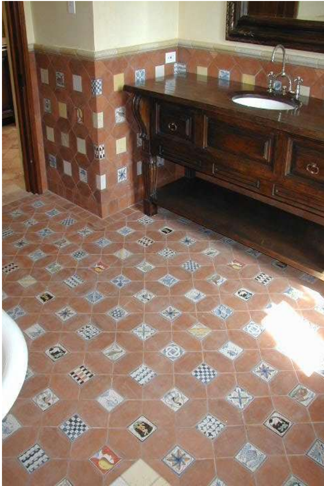
4"x 4" Tivoli decorative tiles inserted between our Unglazed Terracotta 4"x 8" losanges to form a Cassettoni pattern.
