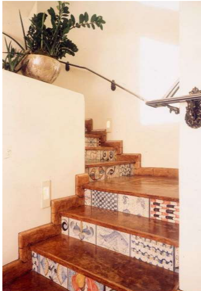
6"x 12" Tivoli decorative tiles used as stair risers underneath these unglazed custom terracotta treads.
