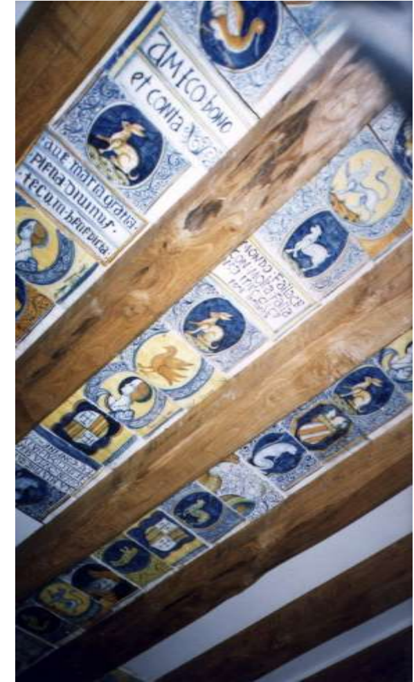
4"x 8" Tivoli decorative tiles inserted between antique wood beams for a wine cellar ceiling.
